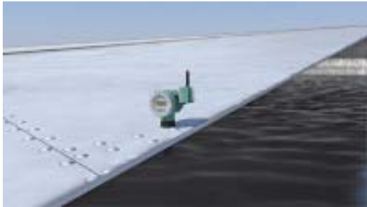
Fig. 3: WirelessHART applications: level measurement
